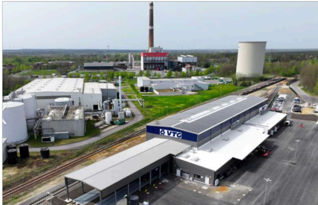
The new state of the art workshop at Grossräschen boasts an impressive maintenance capacity of approximately 2,000 freight wagons per year.
